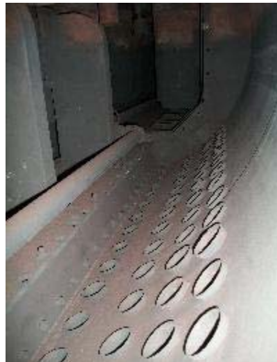
Photo No. 3.29.5 – Boiler No. 3 Steam Drum
