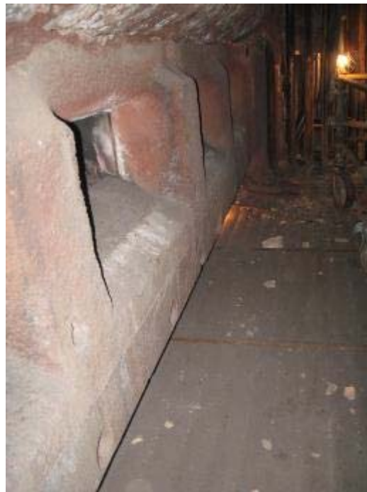
Photo 3.10 – Boiler 5 Front Wall
