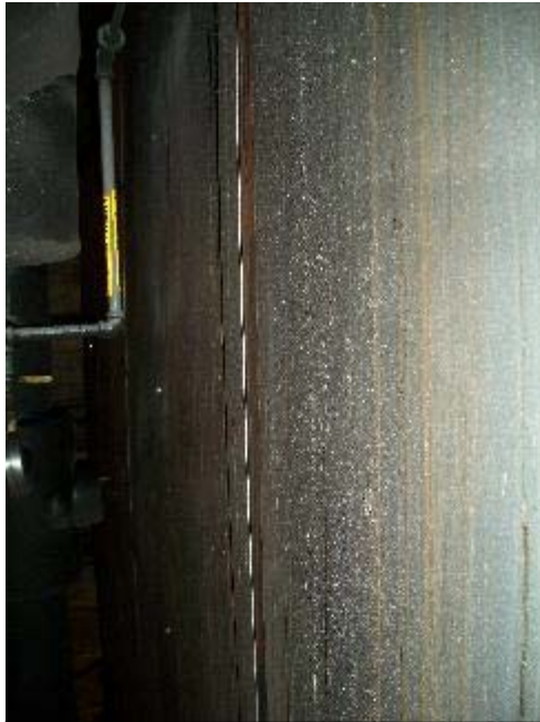
Photo No.3.28.3 – Boiler No. 3 Casing
