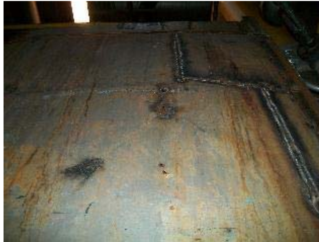
Photo No. 3.28.1 – Boiler No. 2 Casing
