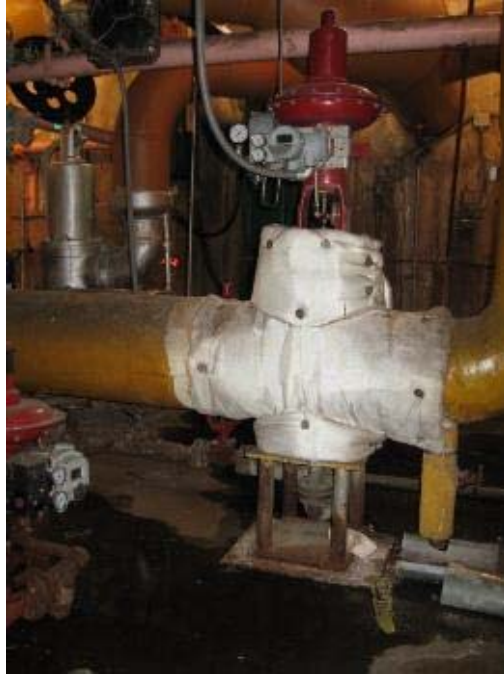
Photo 3.26 – Desuperheater Station
