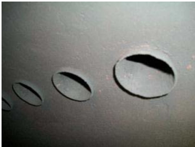
Photo No. 3.29.3 – Boiler No. 3 Mud Drum
