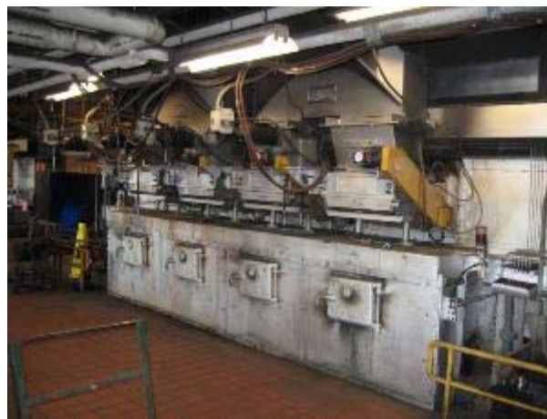
Photo 3.4 – Coal Feeders
