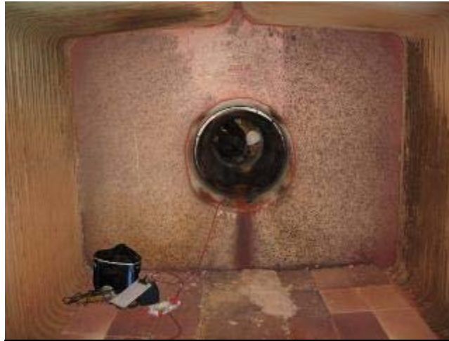
Photo No. 3.29.7 – Boiler No. 3 Furnace
