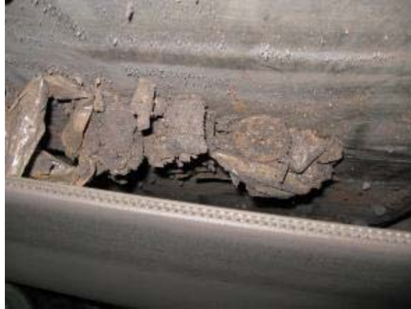
Photo 3.27 – Coal Conveyor Magnet
