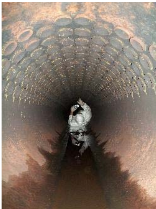
Photo No. 3.29.1 – Boiler No. 2 Mud Drum
