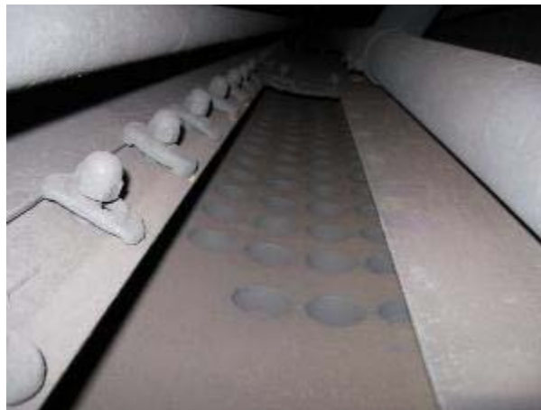
Photo 3.8 – Boiler 7 Steam Drum
