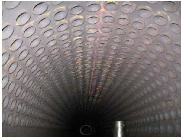
Photo 3.7 – Boiler 7 Mud Drum
