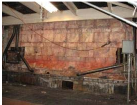
Photo 3.2 – Boiler 5 sidewall & downcomers
