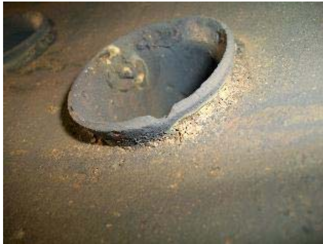
Photo No. 3.29.2 – Boiler No. 2 Steam Drum
