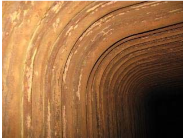
Photo No. 3.29.6 – Boiler No. 2 Furnace
