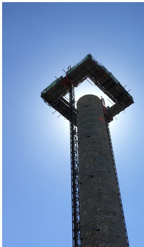
Top/Above: Crews began dismantling the plant's south energy stack in April.
